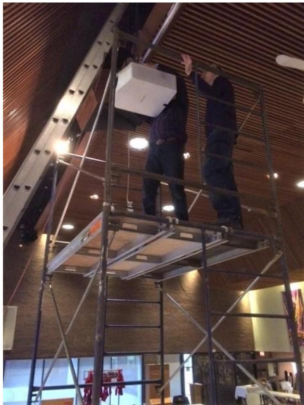
Installing the new projector
