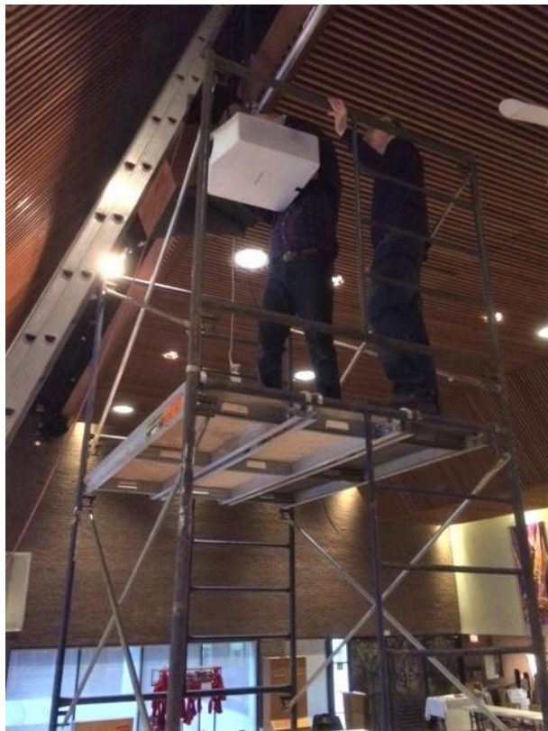
Installing the new projector
